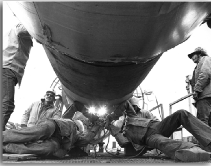
Welders complete final weld for the Trans-Alaska Pipeline, May 30, 1977.
