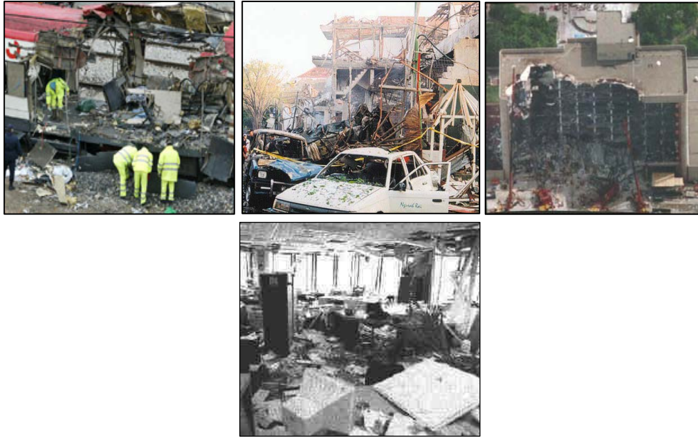
Figure 14 Damage from (clockwise from upper left): Backpack IED, Car-based VBIED, Truck-based VBIED, and Letter Bomb (Source for letter bomb photo: Safecity.com undated)
