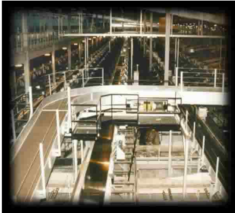
Figure 10 Conveyors at UPS Sorting Facility (Source: Electrical Systems, Inc. undated)
