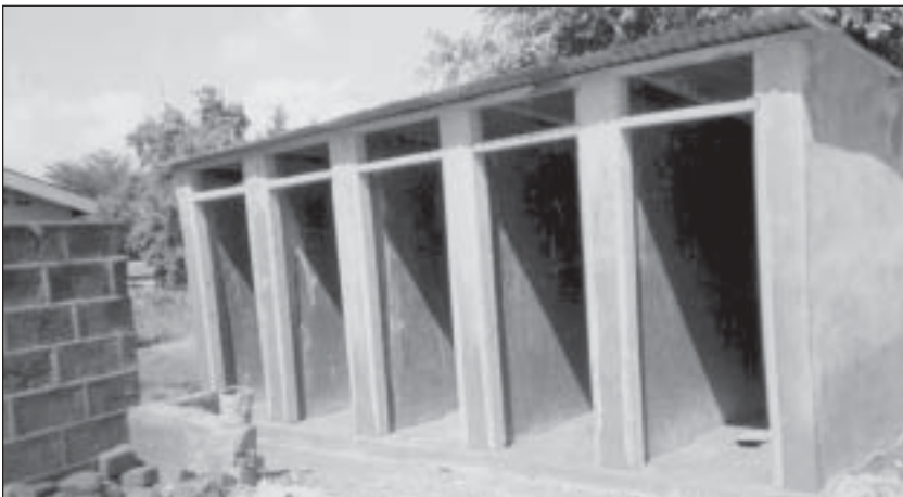
A school latrine construction project nears completion in Kenya.
