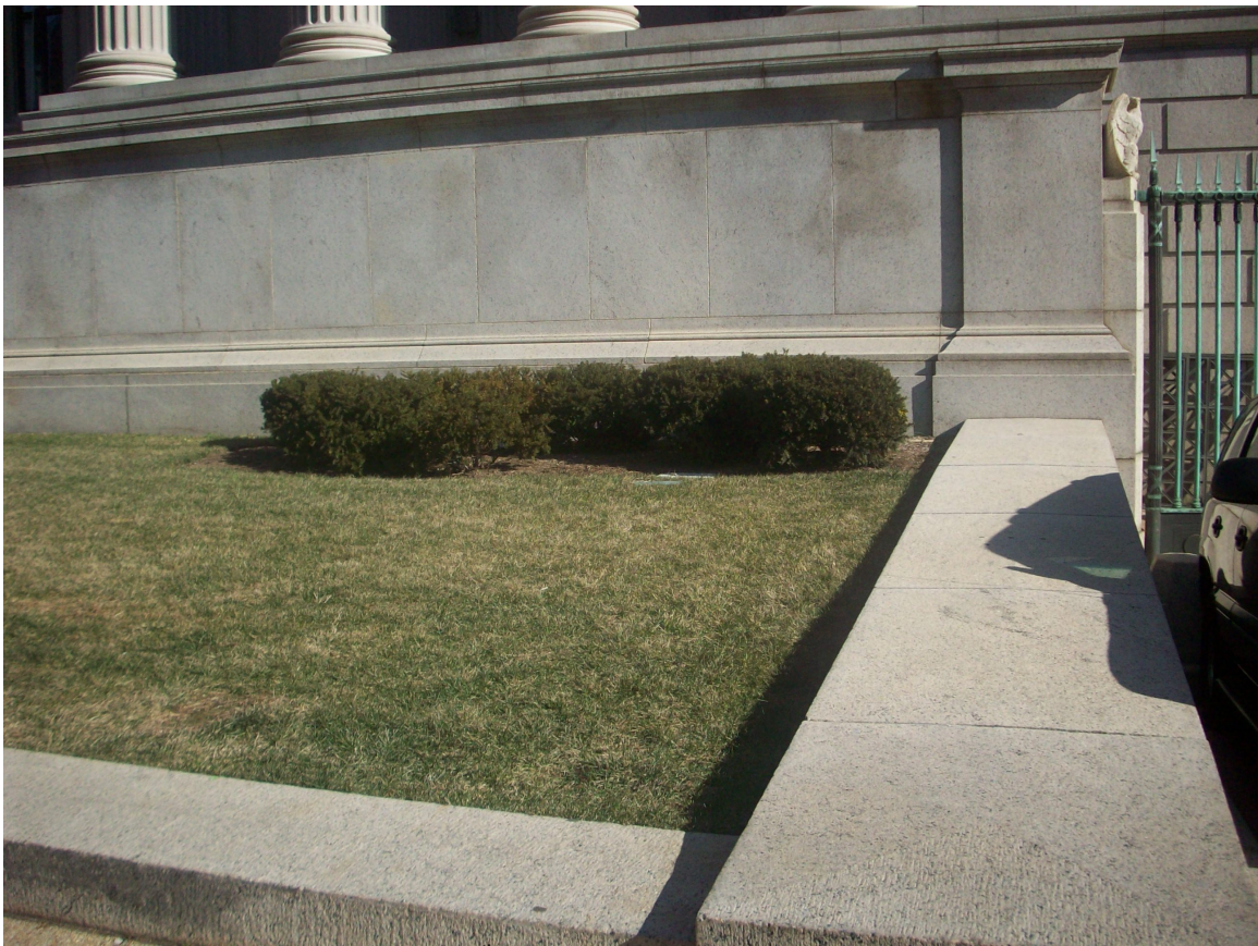
17. View of the north portion of the 9 th Street entrance.
