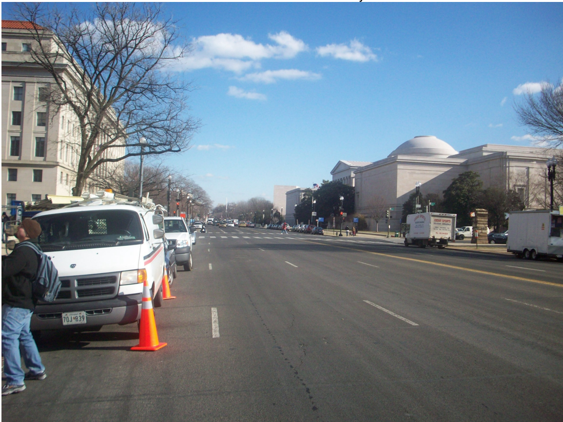
2. View of Constitution Avenue, looking east.
