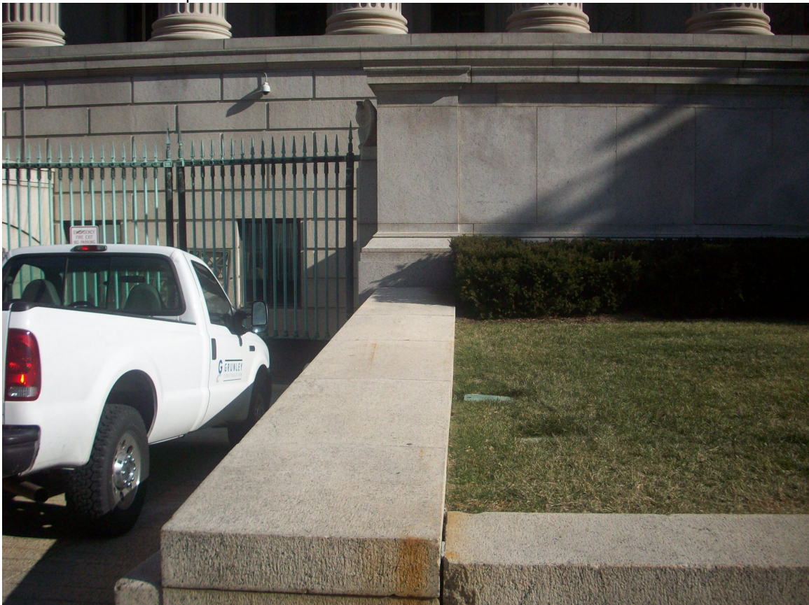
18. View of the southern portion of the 9 th Street entrance.
