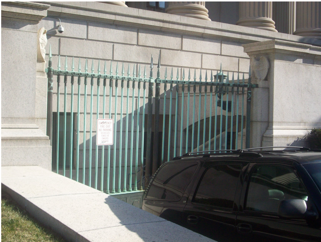
13. View of the 9 th Street entrance, looking from 9 th Street.
