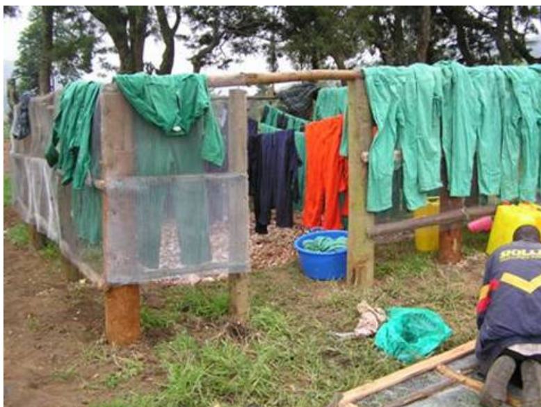
Figure 3. Soak Pit Surrounded by Wooden and Mesh Fencing
