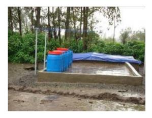
Plastic sheeting and a 3,000 liter tank are used to handle DDT waste water in lieu of an evaporation tank.
