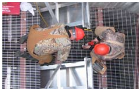
Below: Researchers installing a new lamprey passage structure at a Bonneville Dam fishway.
