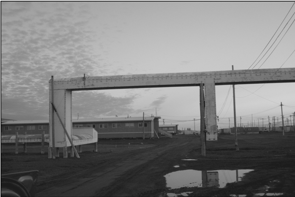
Figure 9. Utilidor in Barrow, Alaska.
