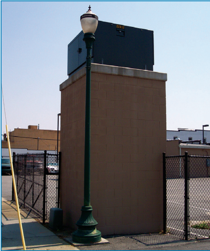
Figure 3-48: Elevated utility box
