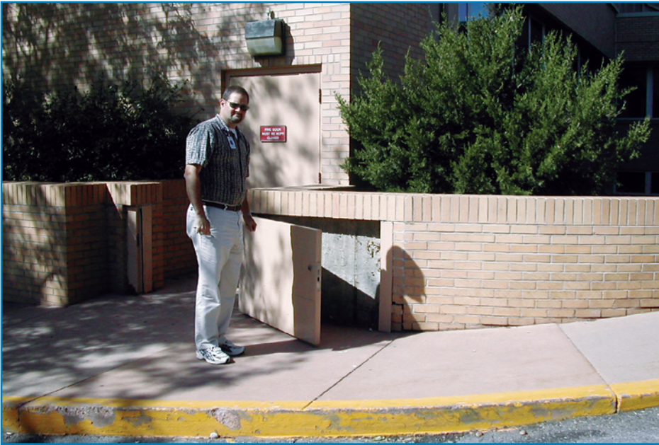
Figure 3-41: Boulder Community Hospital, Boulder, CO, installed this permanently mounted floodgate in a low floodwall; the floodgate swings to the left to keep water away from the mechanical equipment room.
