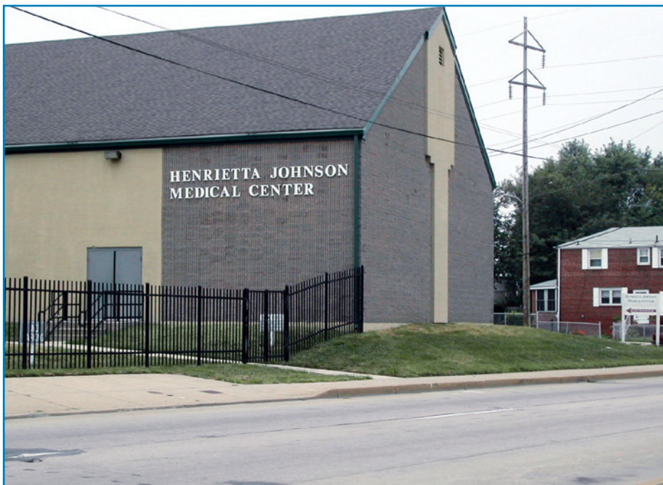
Figure 3-27: Structural fill was placed to elevate the Henrietta Johnson Medical Center above the shallow flood hazard area in Wilmington, DE.
