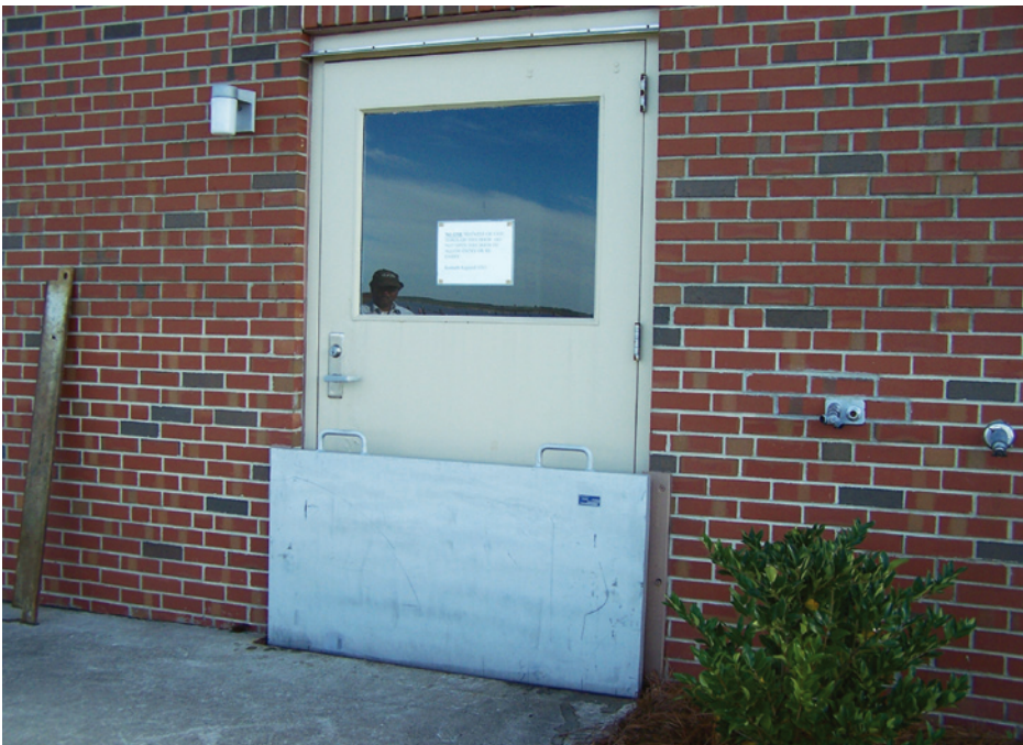
Figure 3-46: Most of the panels can be installed by hand. Note the protective metal strip leaning against the building on the left; normally this strip covers the horizontal channel into which the panel is inserted.
