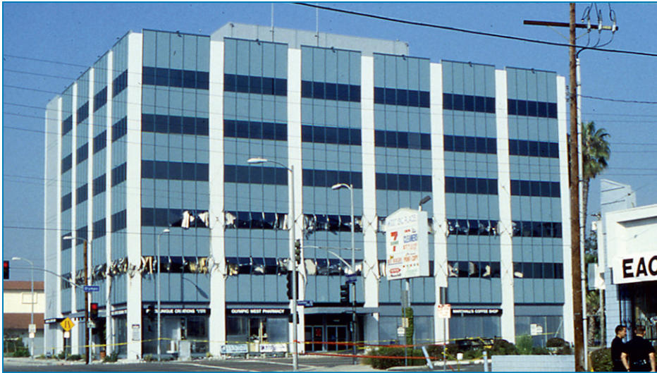
Figure 2-17: A steel frame building with a post-earthquake “lean” to the right, seen particularly at the first floor. Severe damage was found in its beam-column joints and it was later demolished.
