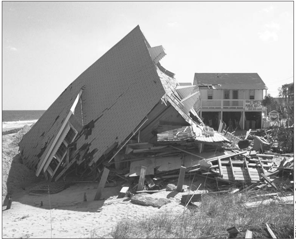
High winds destroyed one house, but left another, that had been elevated, with only minor damage.
