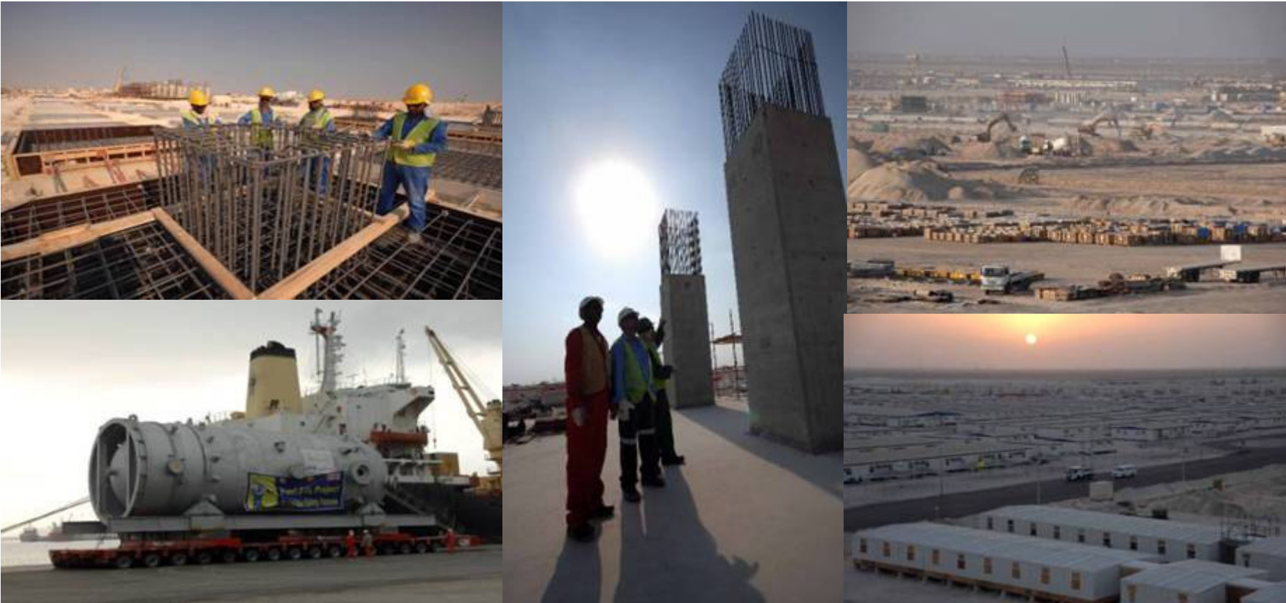
Construction of Pearl GTL at Ras Laffan Industrial City in Qatar
