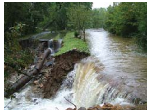
Damage to the city water system in Asheville, North Carolina, following a hurricane in 2004.
