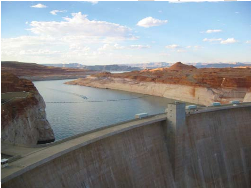
Reduced water levels on the Lake Powell reservoir leave a “bath tub ring” that shows the previous water level. This photograph was taken in July 2004, when the lake was at about 10 million acre feet (120 feet below full, 40 percent of capacity). In April 2005, the lake level was even lower, about 8 million acre feet or 33 percent of capacity.
