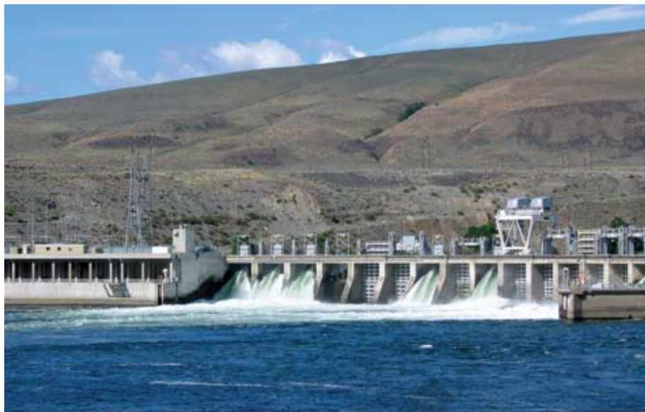
Hydroelectric dam in the Northwest.
