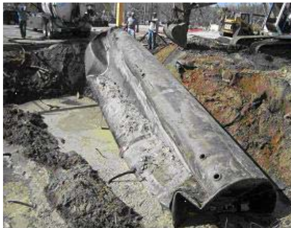
Figure 3 - Storm-damaged UST in Mississippi. (Source: MDEQ)
