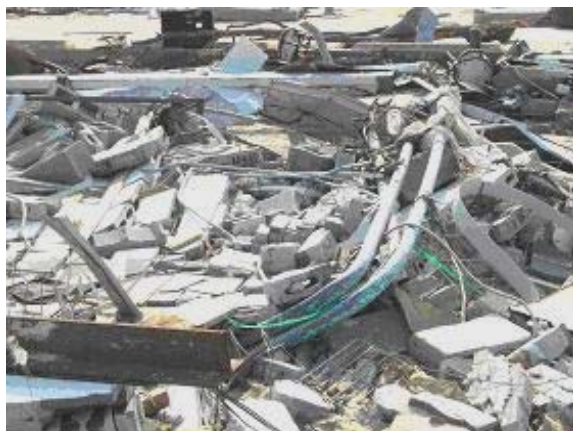
Figure 4 - Twisted UST vent lines in a debris pile. (Source: MDEQ)
