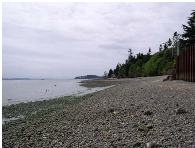
Figure 4-5 -A sheet pile wall, right, contains contamination impacting the Suquamish Tribe from the Wyckoff-Eagle Harbor site (OIG Photo)
