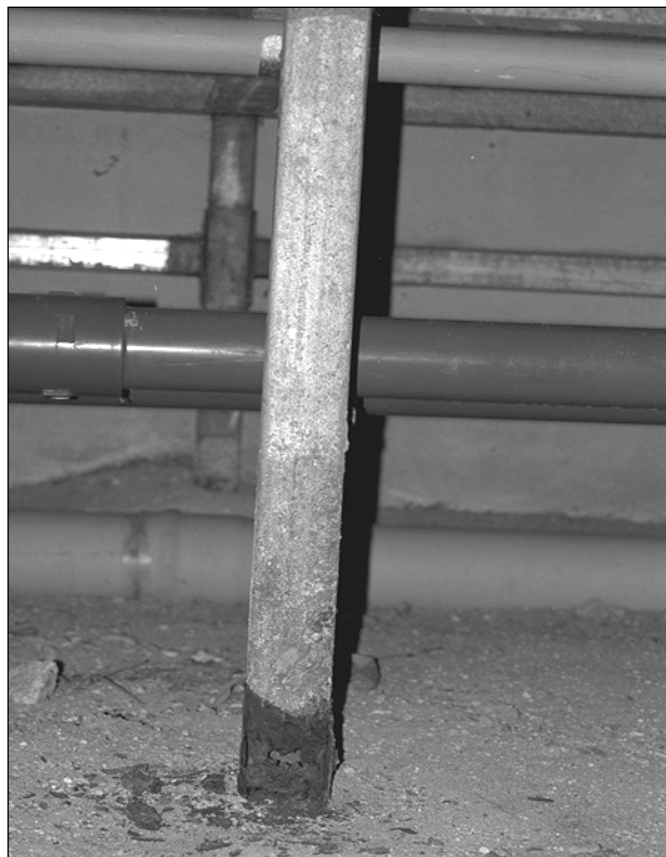
Foundation Piers in New Ebeye Hospital
