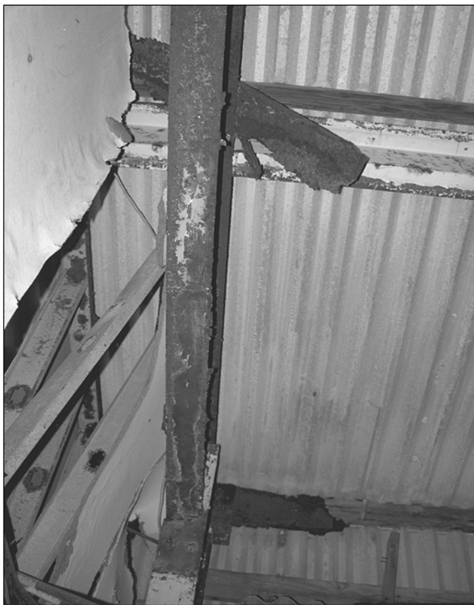
Roof Beams in Existing Ebeye Hospital
