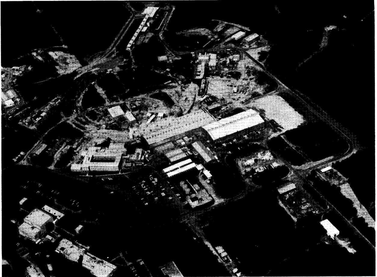
Figure 4. Aerial photo of Brookhaven's Alternating Gradient Synchrotron. This proton accelerator lies in a tunnel under the circular mound at top left.
