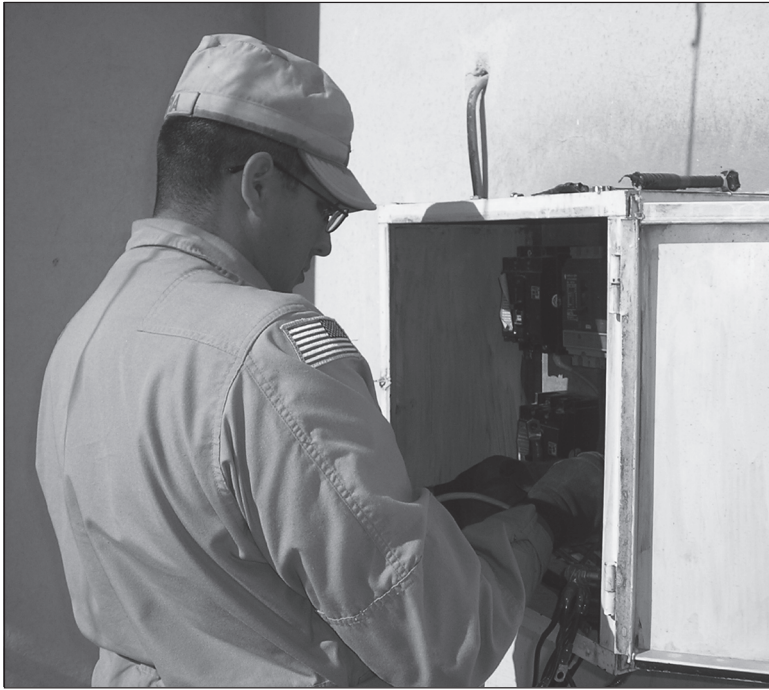
A Soldier works at troubleshooting an electrical fault.
