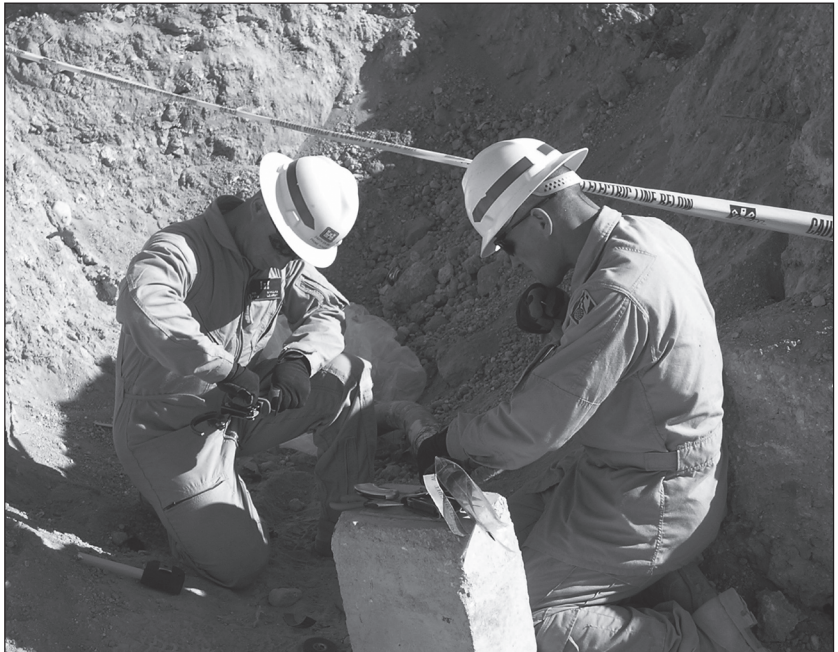
Soldiers splice a medium-voltage distribution cable.
