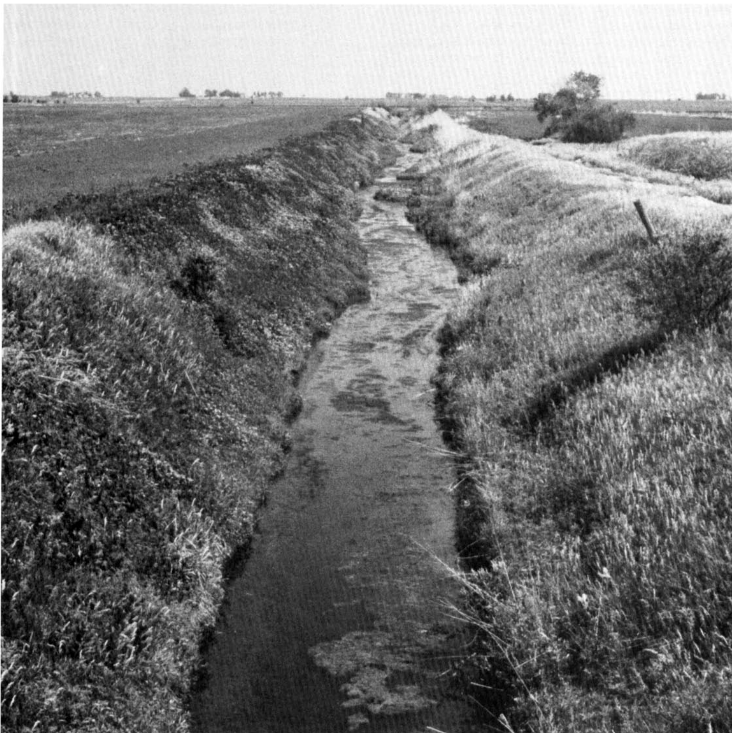
Figure 8.—A drainage ditch in an area of Canisteo silty clay loam, 0 to 2 percent slopes. Drainage ditches provide outlets for subsurface tile drains.
