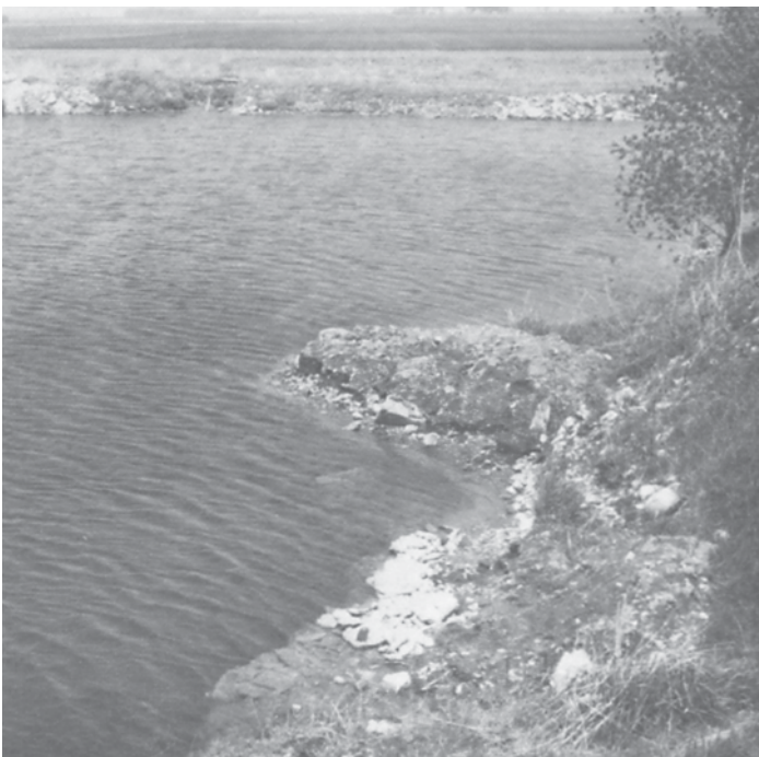
Figure 14.—Limestone quarry in Faxon soils needs pumping in order to excavate limestone.
