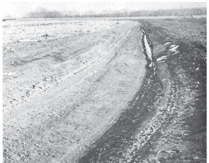
Figure 9. —Two parts of the Vesser-Lawson-Nodaway association. Top: Before the flash flood in September 1965 this area was in beans and pasture. Bottom: Recently constructed drainage ditch.
