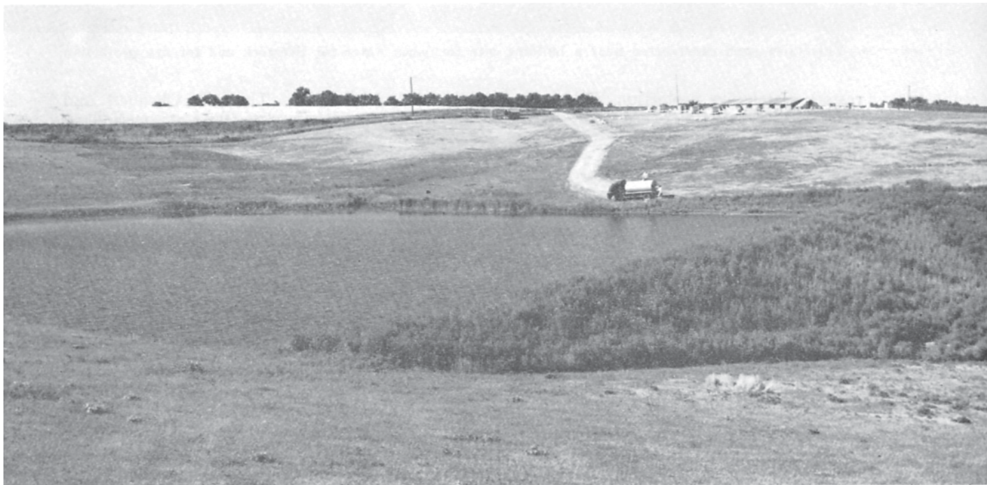
Figure 19.—A farm pond that is used to water livestock in a pasture. The backslope of the earthen dam to the right is well seeded. Shelby and Clarinda are the dominant soils in the background.
