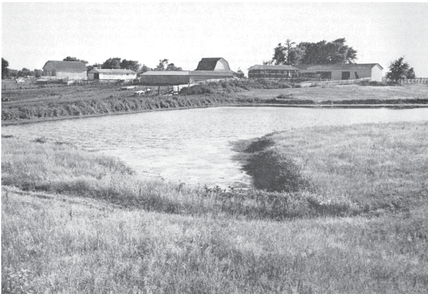
Figure 20. —This farm pond constructed near a building site furnishes water for livestock and for fire protection.
