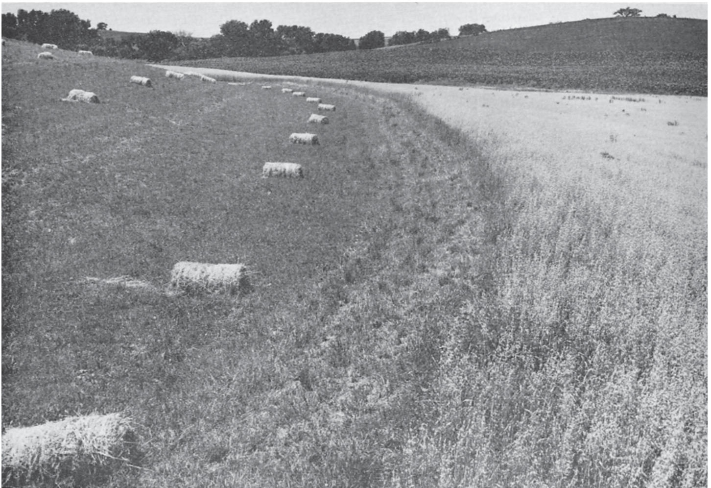
Figure 10.—A diversion terrace built at the base of an upland slope so as to protect Colo silty clay loam, 2 to 5 percent slopes, from local runoff.
