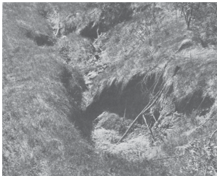
Figure 2.—Limestone sinkhole in road ditch in the Dinsdale-Klinger-Maxfield soil association.
