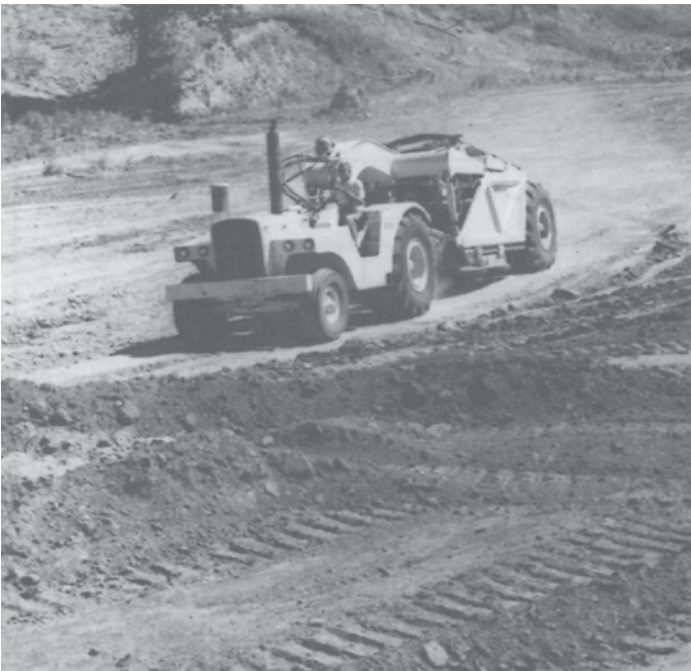
Figure 29.—Farm pond being constructed on Lindley soils.
