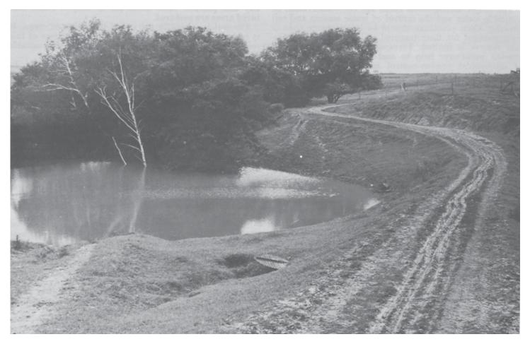
Figure 13.—Farm pond used to stabilize a gully and to provide a wildlife and recreation area.
