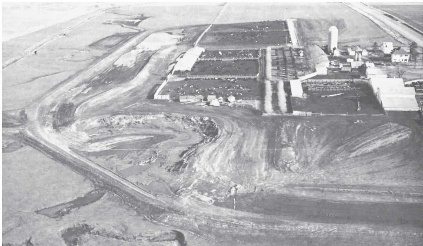
Figure 6. —Pollution-control structure designed for cattle-feeding operation.
