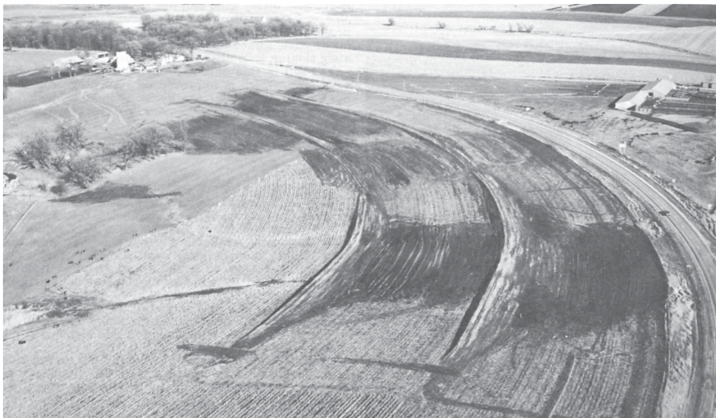
Figure 14. —Parallel terraces provided with tile outlets on Tama soils. The backslope of the terraces is seeded to grass.
