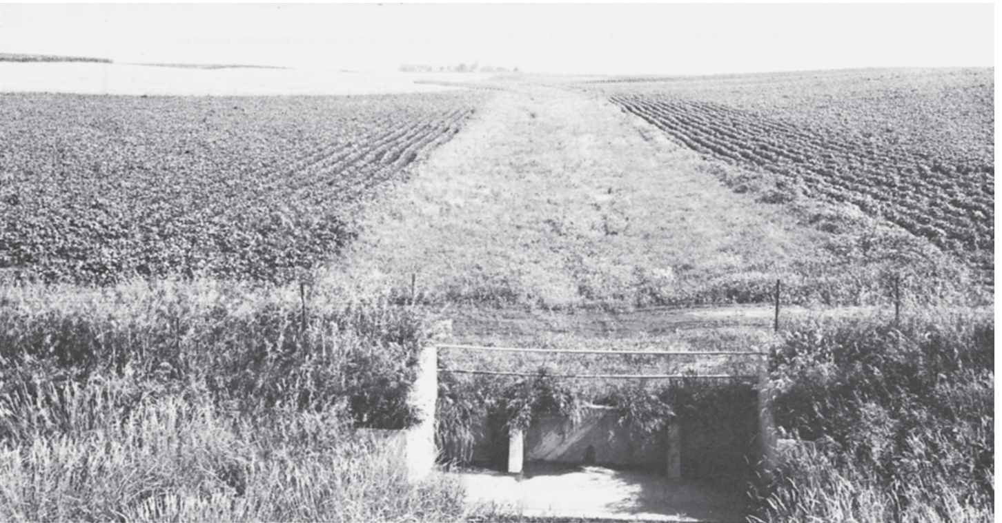
Figure 12. —Grassed waterway, drop structure, and tile outlet on Sawmill-Garwin silty clay loams.
