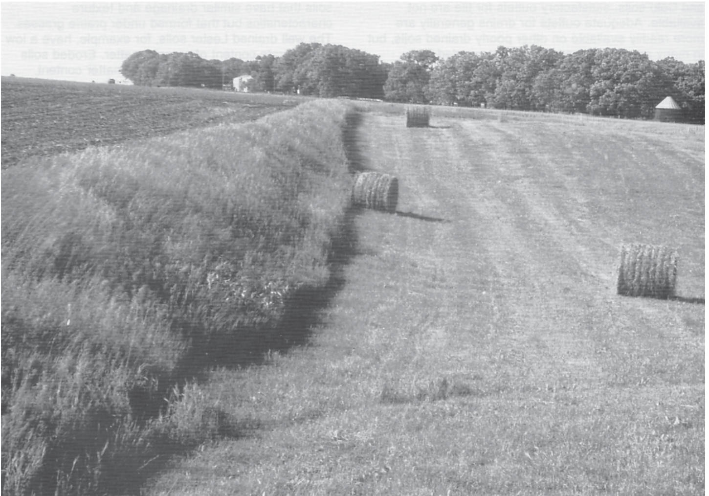
Figure 17. —This water- and sediment-control basin helps to control erosion and sedimentation in the waterway. Bromegrass grown in an area of Clarion loam, 5 to 9 percent slopes, moderately eroded, below the structure provides additional protection from runoff and erosion.
