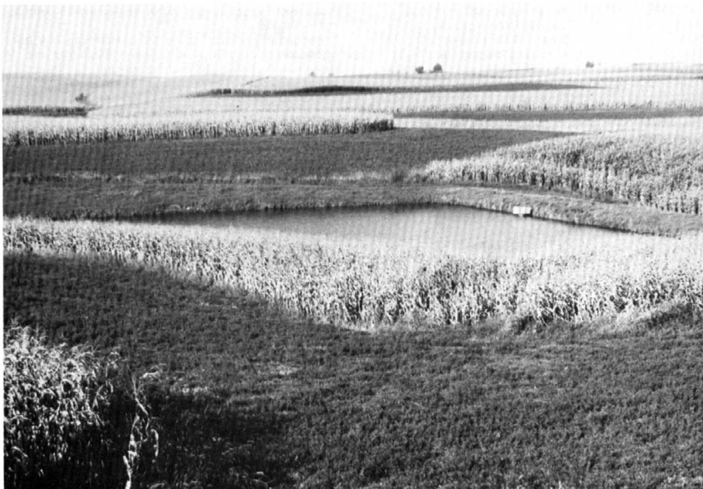
Figure 10.—Erosion control structures are commonly used on steep slopes of the Fayette soils to control gully erosion. Some of these structures provide water for livestock and recreation.
