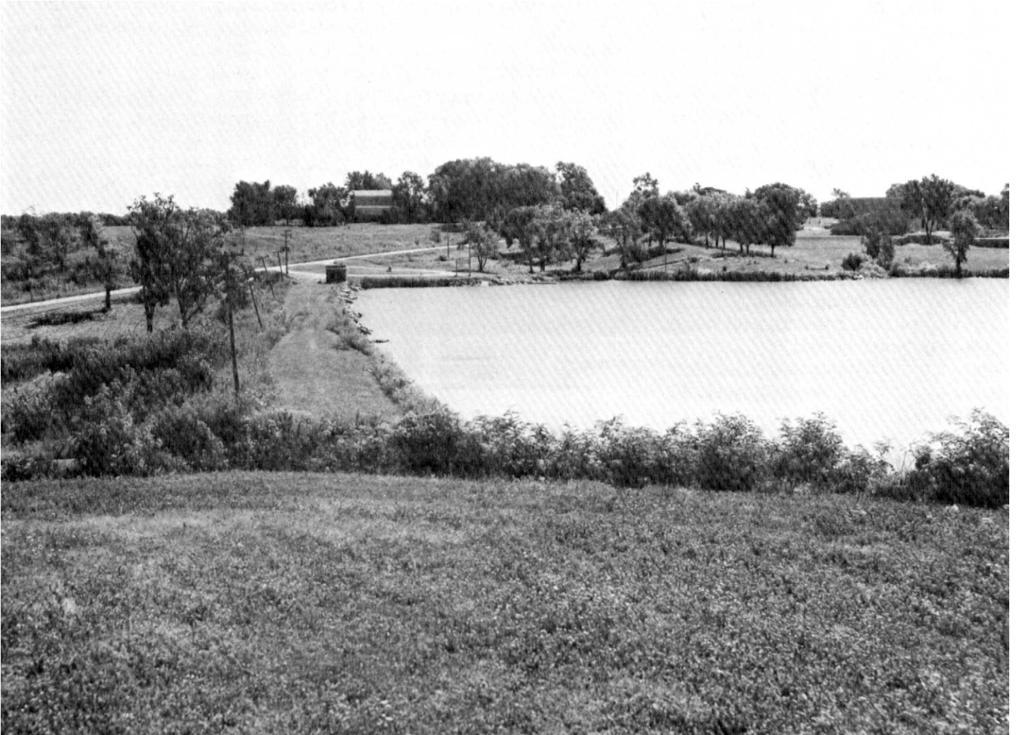
Figure 10.—A water-control structure that protects cropland in the valley of the Fox River from flooding and provides a source of water for the city of Bloomfield.
