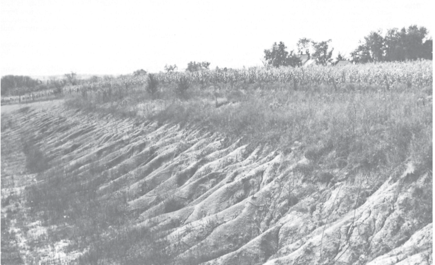
Figure 8.—Road cut exposing the buried soil in which Clarinda soils formed.
