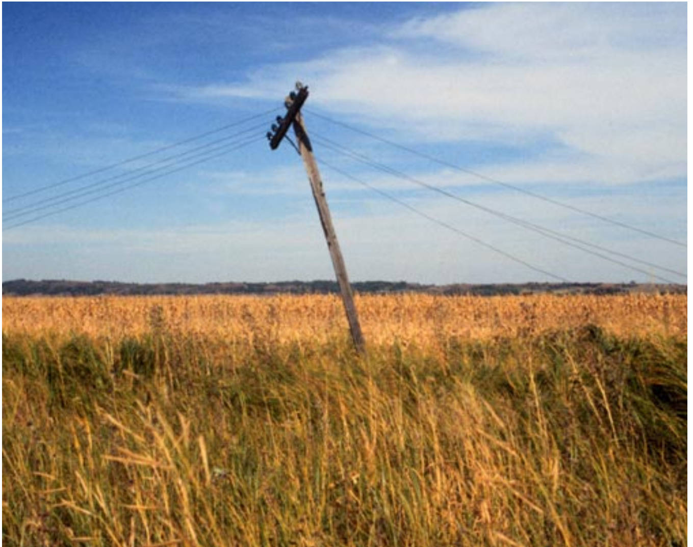
Figure 15.—An area of Luton silty clay, 0 to 1 percent slopes, rarely flooded. The high shrink-swell potential can damage roads, building foundations, and utility lines.
