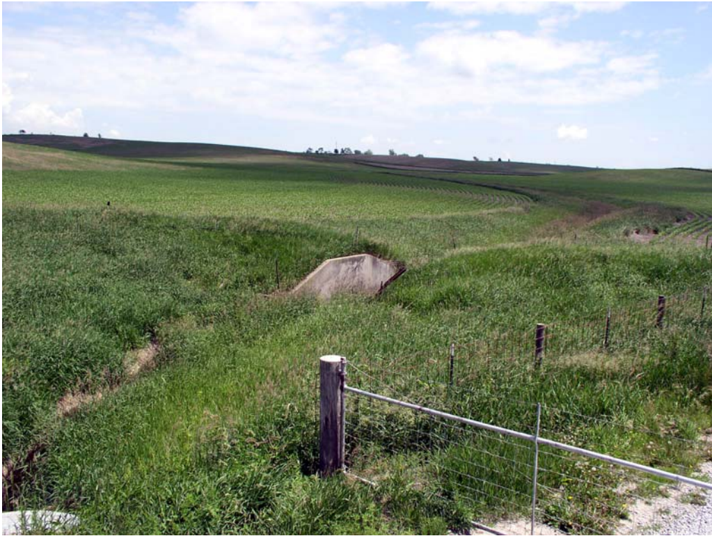
Figure 12.—Drop structures, grassed waterways, and contour farming help to prevent further erosion in an area of Colo-Ely complex, 2 to 5 percent slopes.
