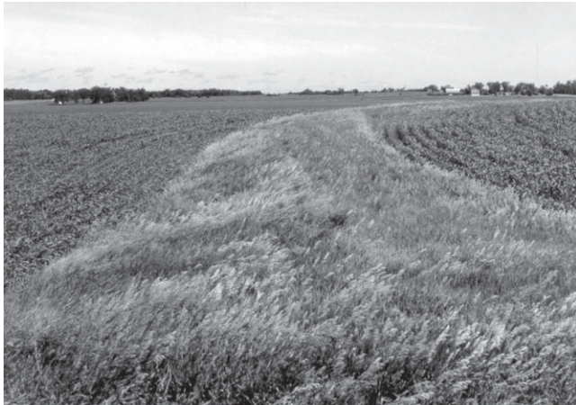
Figure 10. —Grassed backslope terraces constructed across the slope help to control water erosion in an area of Clarion loam, 5 to 9 percent slopes, moderately eroded.
