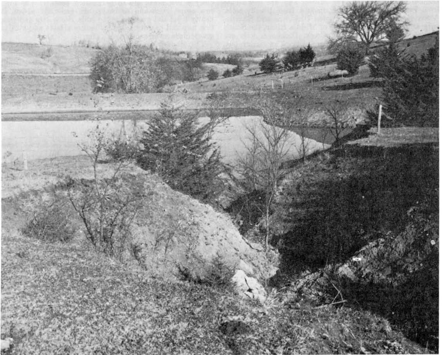
Figure 4.—Gully control structure in the Sharpsburg-Ladoga-Shelby association.
