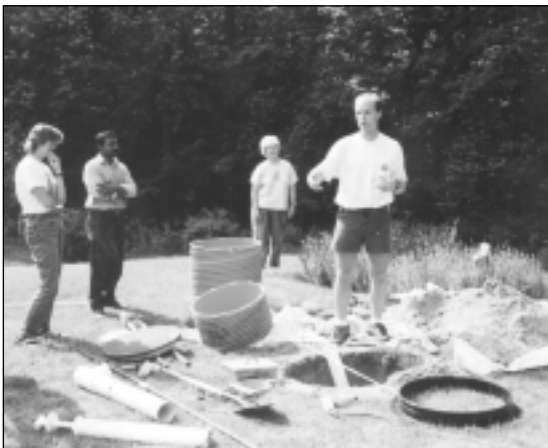
The NODP II project in the town of Jericho involved a heavy emphasis on public education, including the installation of effluent filters and risers for a septic tank.
