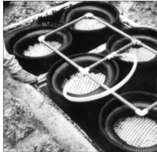
Demonstration projects serve as testing grounds for phosphorus removal technologies. Shown here are biofilter baskets and the distribution system of a site at the Benzie County, Michigan NODP project (above) and a continuous feed cyclic reactor at the Florida Keys Onsite Wastewater Nutrient Reduction Systems Demonstration Project in the lower Florida Keys (right). Benzie County photo courtesy of Bill Crawford
