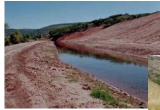
Repaired ditch prior to reseeding
