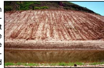
Repaired area above ditch
