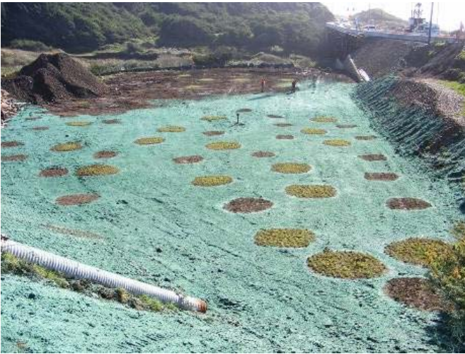
Rock Creek restoration area, north of Florence, OR. Circles were planted densely with plugs of violets or nectar species. Area in between was hydro-mulched with fescue, yarrow, and violet seed.
