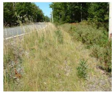
Seeding of shoulder after repavement of road
