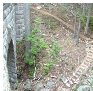
Planting with rock steps along abutment
