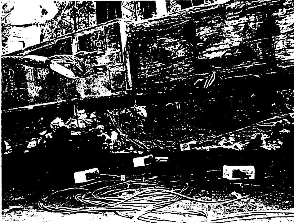
Figure 4. Placement of DCDT's under midspan of skidder bridge.
