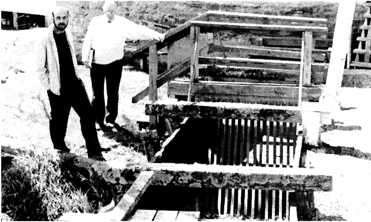
Figure 4 - Existing Timber Flume, Pedestrian Bridge, and Trash Screen.
