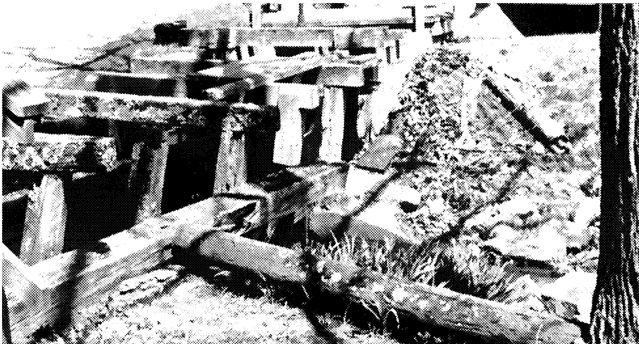
Figure 6 - Existing Timber Flume, Waste Gate and Stone Spillway.
