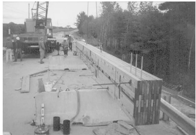
Figure 7—Bridge components were preassembled into mini-modules at construction site.
