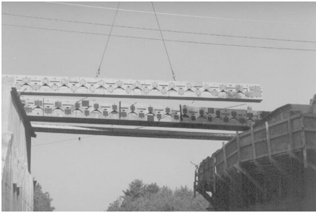
Figure 8—Mini-modules were lifted by crane onto concrete abutments.
