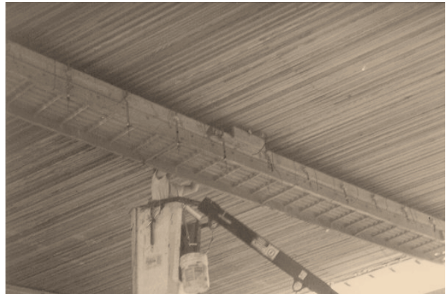
Figure 16—Displacement transducer used to measure bridge deflections in load tests 1 and 2.
