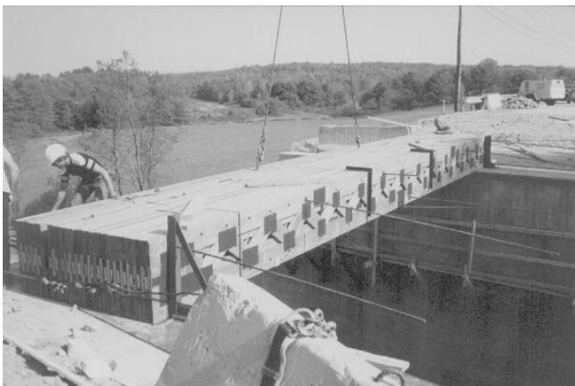
Figure 9—Modules were placed side by side to form bridge width.
