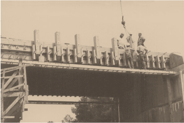
Figure 12—Installation of rail system.
