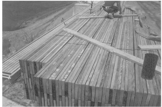
Figure 10—Modules were staggered to accommodate 11.5° skew.
