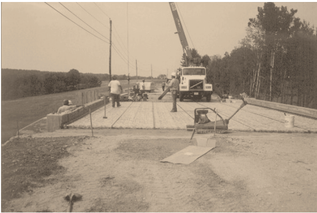
Figure 13—Bridge after installation of waterproof membrane.
