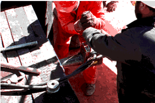
Figure 7—Stressing bars were hammered through the final deck section.
