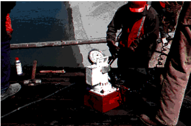
Figure 8—Hydraulic jack with built-in ratchet (top) and electric pump (bottom).
