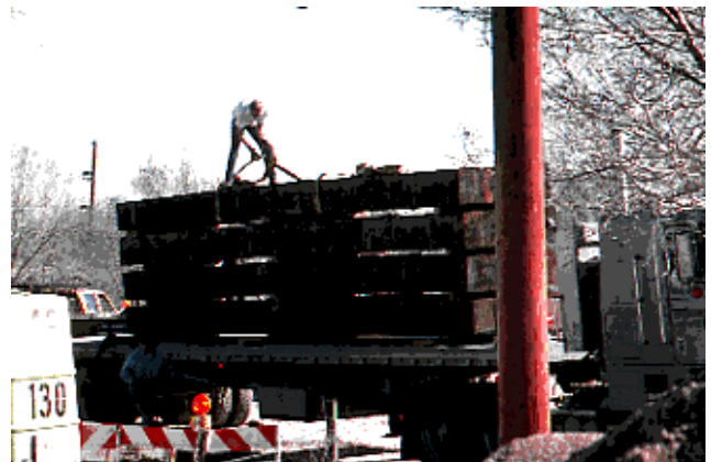
Figure 5—Bridge superstructure delivered in four preconstructed sections banded with steel straps.
