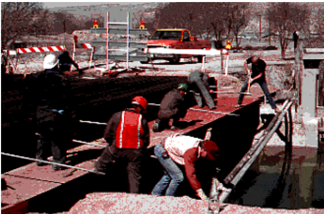
Figure 7—Stressing bars were hammered through the final deck section.
