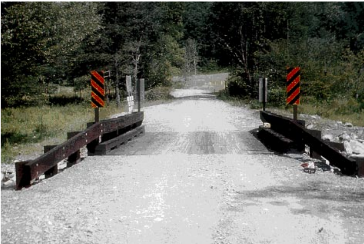
Figure 10—Completed Little Salmon Creek bridge.
