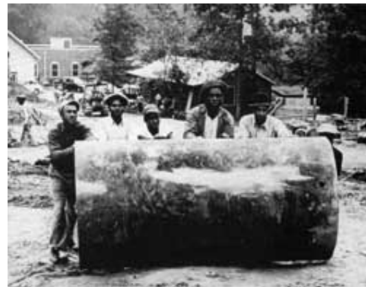
Construction work gang rolling caisson toward Clinical Center excavation site.
