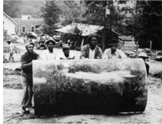
Construction work gang rolling caisson toward Clinical Center excavation site. (Courtesy of the National Library of Medicine.)
