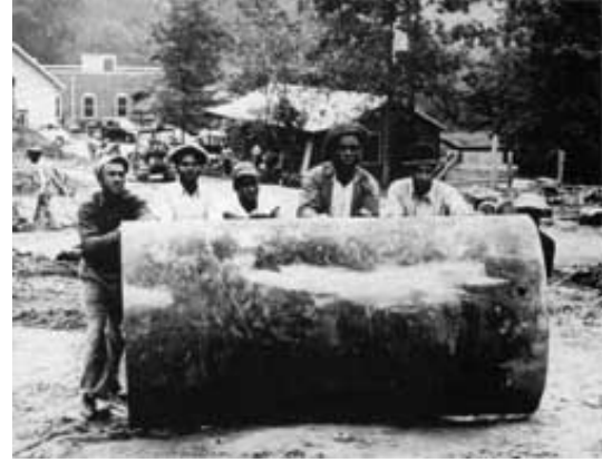
Construction work gang rolling caisson toward Clinical Center excavation site. (Courtesy of the National Library of Medicine.)
