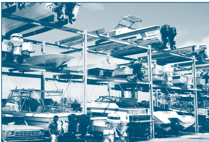
The San Juan Bay Marina in Puerto Rico provides dry stack storage.
