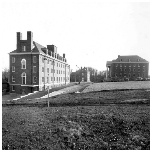
Buildings 1-3 completed Office of NIH History
