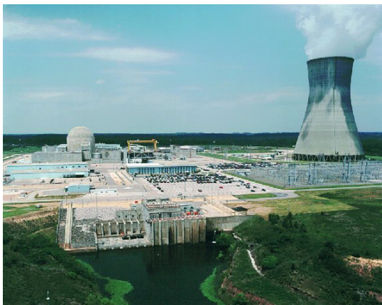
Shearon Harris Nuclear Power Plant.
