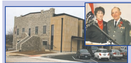
The last major FEMA-funded project from the May 2003 tornado that hit Pierce City was completed this year. The Ray Carver Building was renovated at a cost of more than $3 million. It is now home to Clark Community Mental Health and 50 employees.
