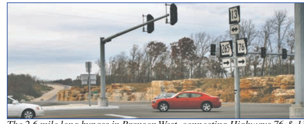
The 2.6 mile long bypass in Branson West, connecting Highways 76 & 13 opened to traffic in late October. Congressman Blunt secured funding to pay for the improvements.
