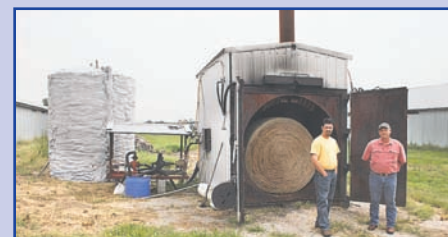
The Youngblood poultry operation near Diamond is using a non-feed, hay-burning furnace to heat six houses. The Youngbloods hope to save thousands of dollars in heating costs with their new innovation which is finding interest from other growers.
