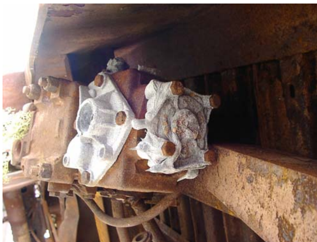
Figure 6-1. Air Brake Valve Found 20+ m [66+ ft] from Fuel Spill Site (Note Only Partial Melting at This Location)
