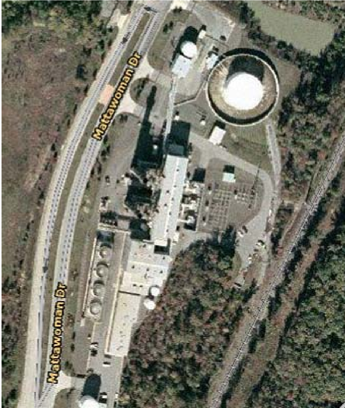
Figure 3 – Aerial Photo Showing Panda Brandywine Site (Source: Mapquest.com 2007)
