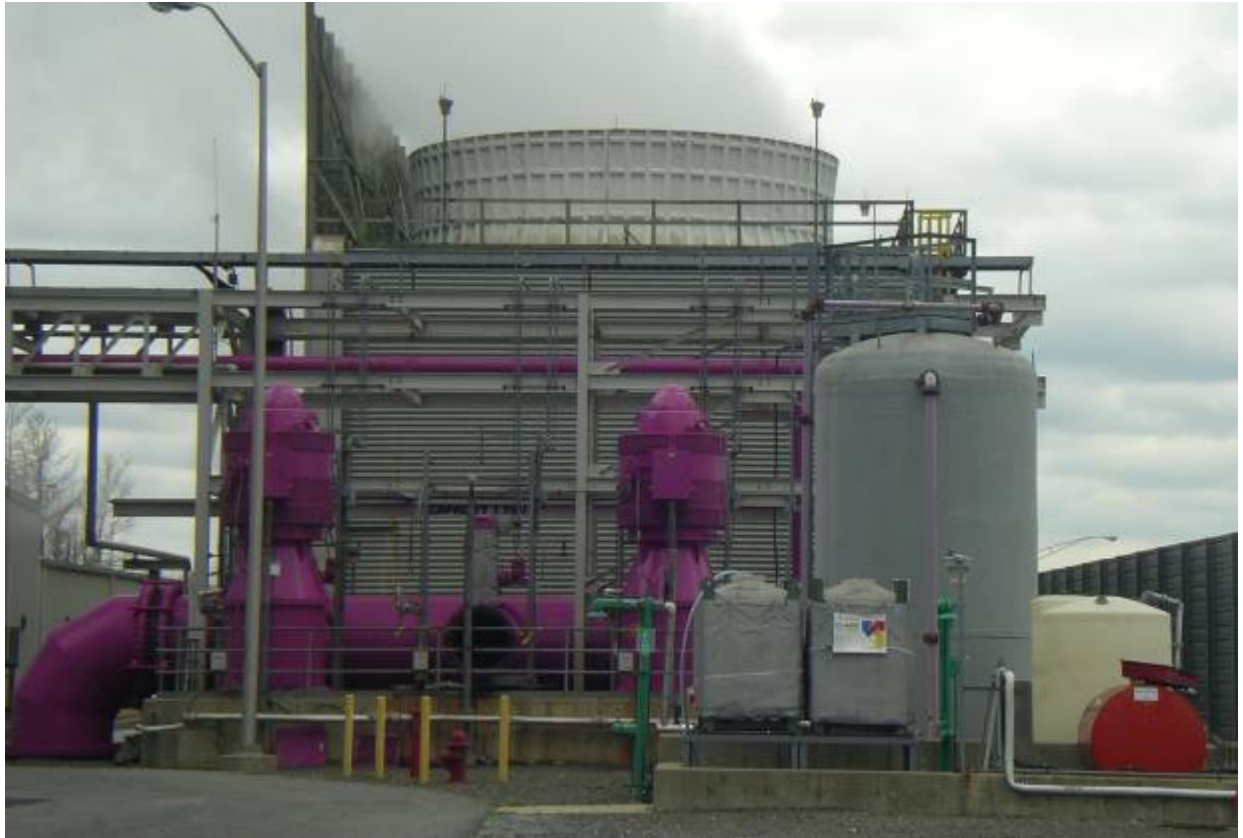
Figure 1 – Reclaimed Water Pipes and Pumps Painted Purple (Source: Veil 2007)
