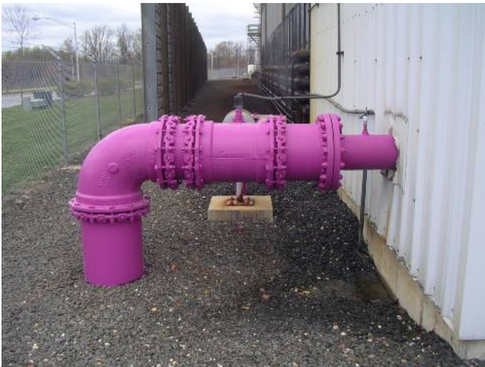
Figure 5 – Reclaimed Water Line Entering Cooling Tower (Source: Veil 2007)
