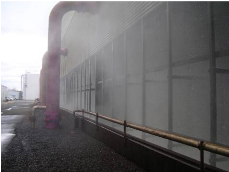
Figure 9 – Reclaimed Water Falling through Cooling Tower and Forming a Mist (Source: Veil 2007)
